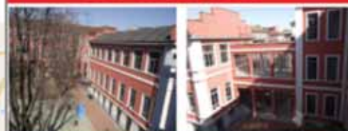
LOWER SECONDARY SCHOOL CIRESOLA 1920 - Renovation 2006
